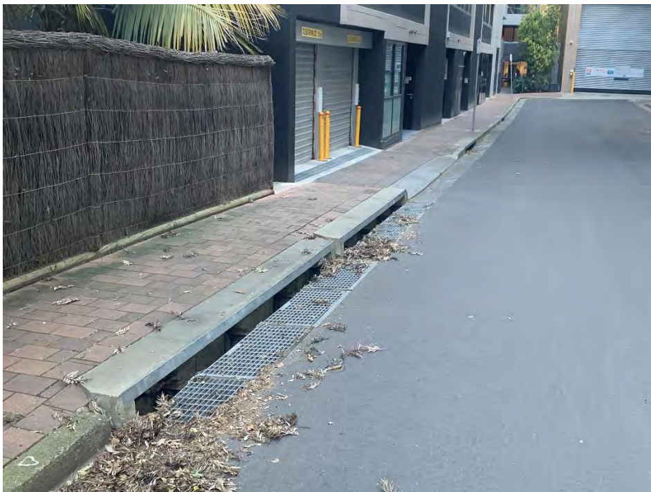
Photo consisting of stormwater pit with 2 x 3.6m lintels within Harnett St
